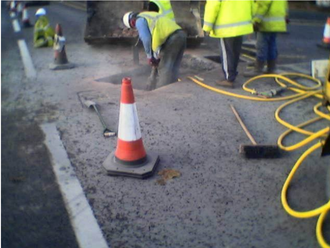
Figure 1: A Pneumatic Drill Operator
